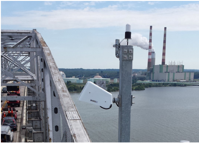
Different Road Weather Stations Source: MDOT
