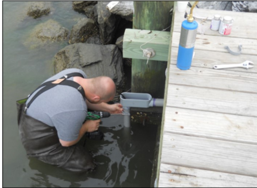
Installing the Conduit for the Orifice Line – St. Mary's County, Maryland
