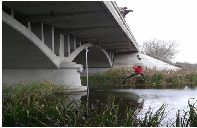
Figure 5. Specially-trained climbers have performed the installation on bridge pillars
