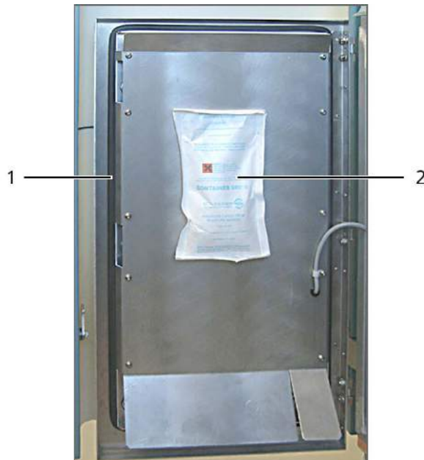
Fig. 30: Air dehumidifier bag (2) and rubber seal (1).
