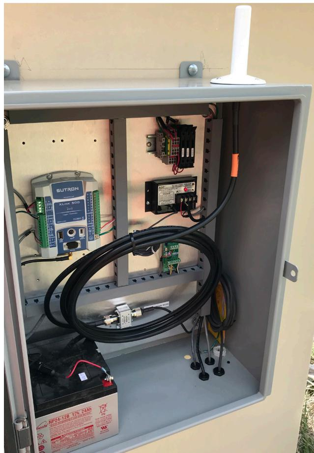
An open NEMA-4 enclosure containing a complete set of equipment, including the SUTRON XLink 500.
