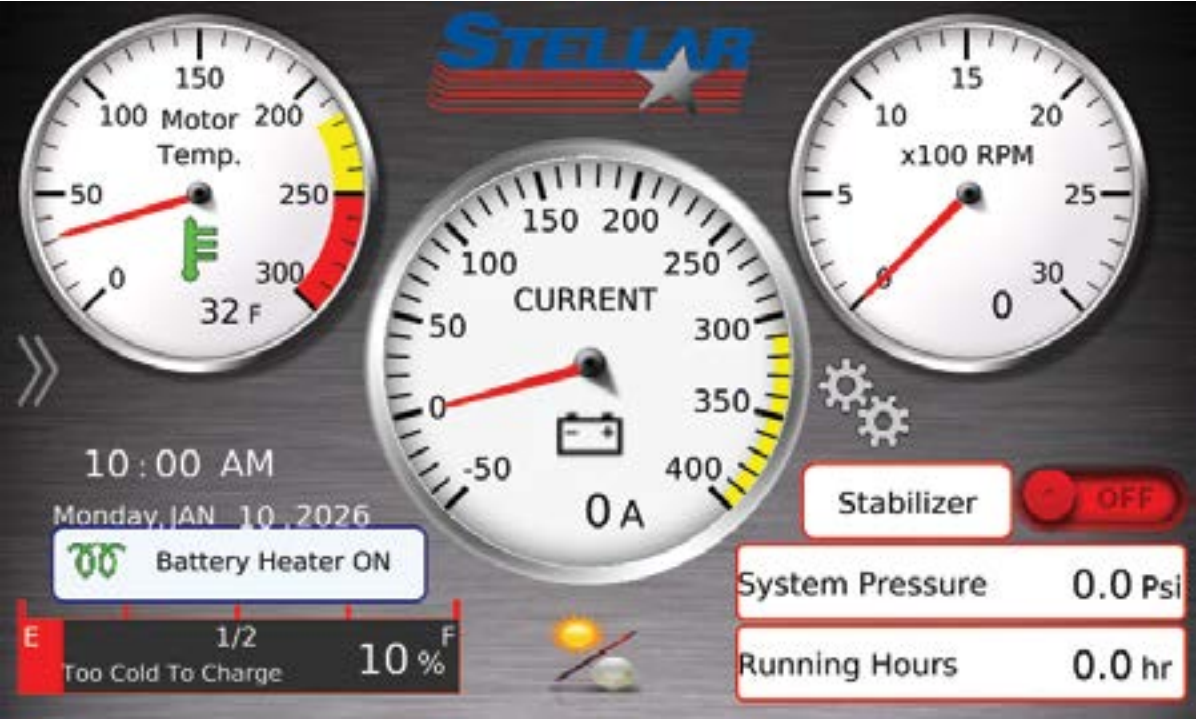
Figure 13: Battery Heater Enabled - Display Screens
